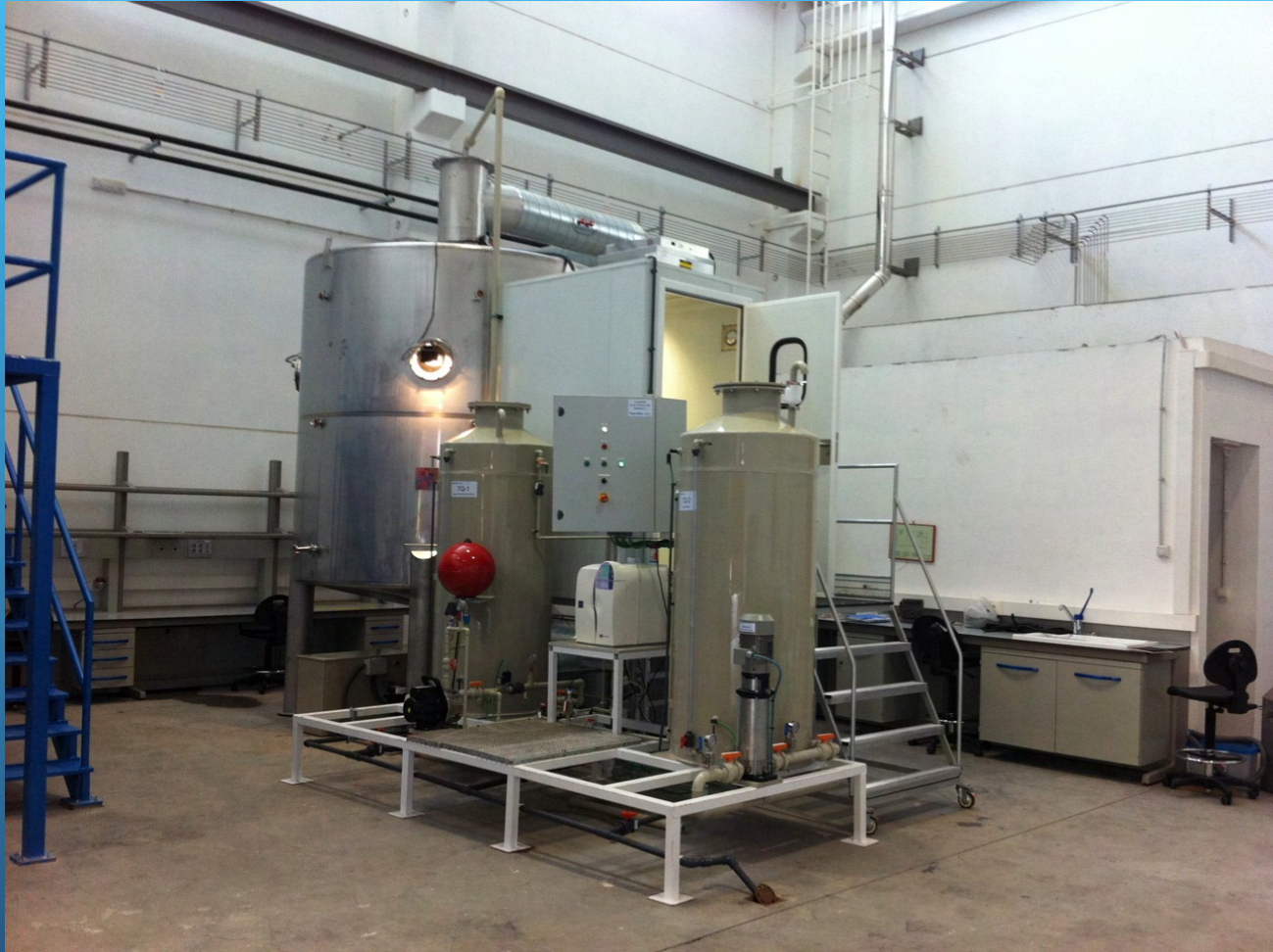
Self-cleaning installation for dispersing engineered nanoparticles
